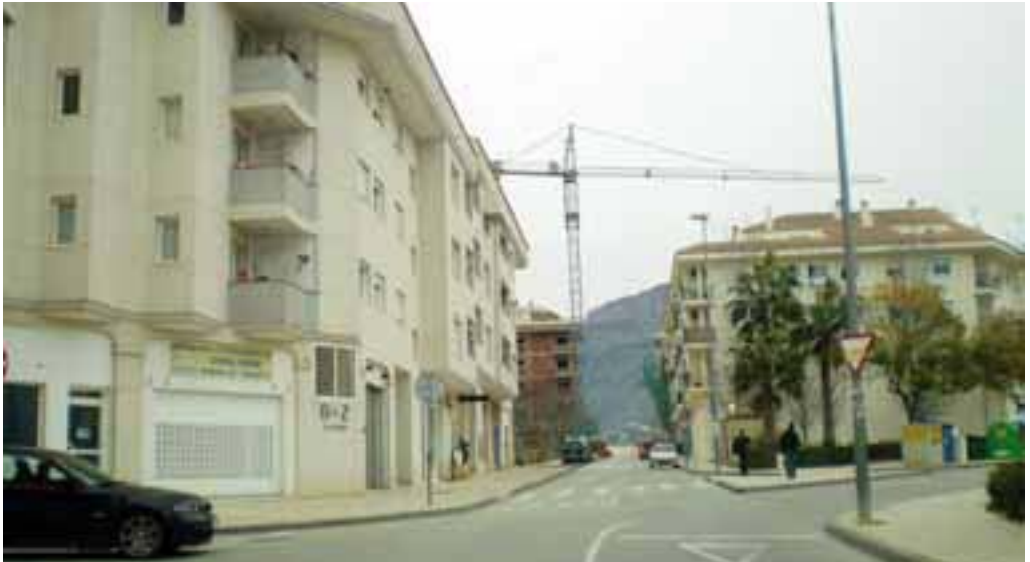
Flats in construction - Barrio de Garganes
